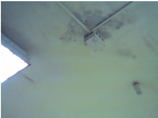
Fig. 3 Temperature sensor – installation and communication channels
