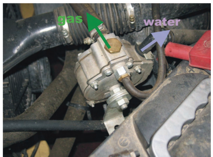
Fig. 11 Position of the pressure reducer in engine compartment
