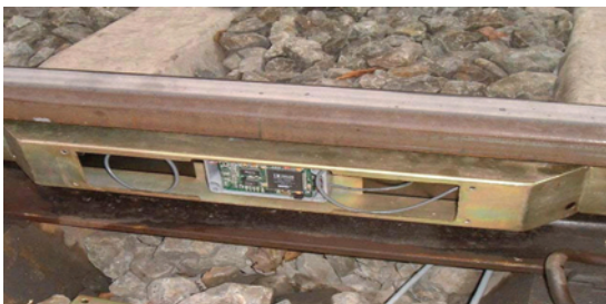
Fig. 7 Measurement device in protective box; sensors are on the left and on the right.
