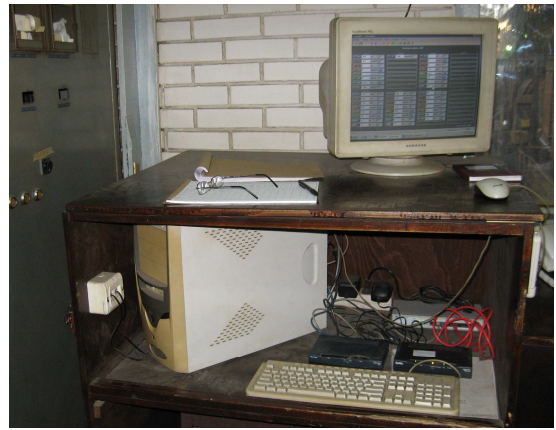
Fig. 3. PC workstation in the converters plant control room
