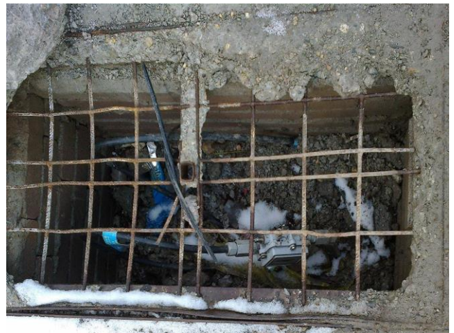
Fig.4. Cable chamber
