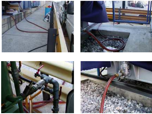
Fig. 1. Connecting the transformer with device by hoses
