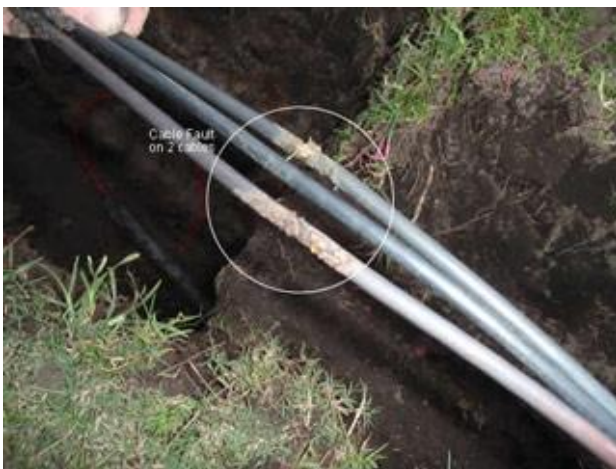
Fig.2. Cable fault - two cables
