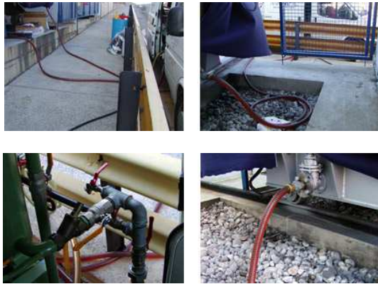
Fig. 1. Connecting the transformer with device by hoses
