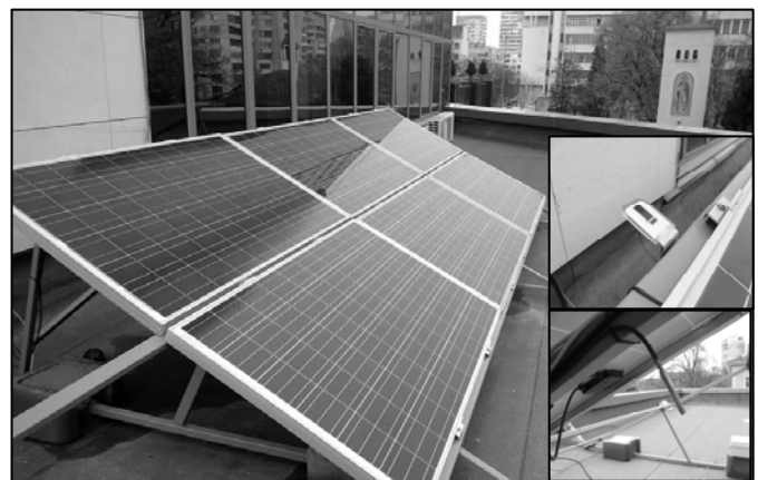
Fig. 3. PV-central on the roof of BFU.
